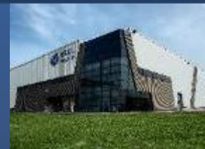
New GTF engine facility, Bet Shemesh
