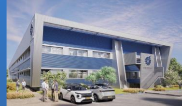
New small engine facility
